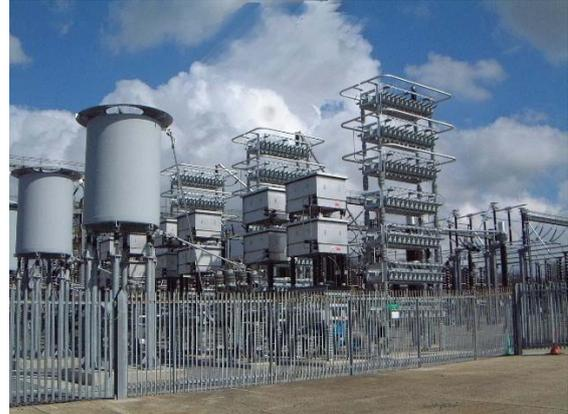
400kV Filter Resistors
