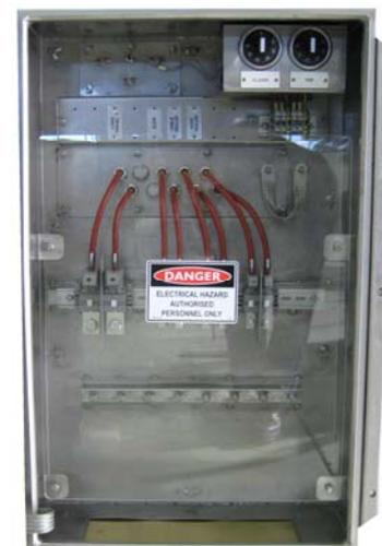
IP56 cable termination compartment showing thermostats, high temperature cable, earthed brass gland plate, cable sheath termination bar, perspex shield, and resistor labels
